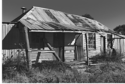
Building between Hill End & Sofala Accepted John Workman
